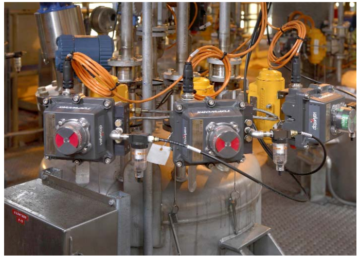
Installation of Valvetop DXPs with FOUNDATION Fieldbus at Eastern U.S. chemical plant
